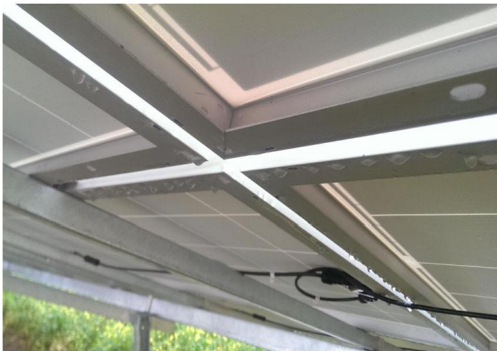
Figure 7. Underside of a Solar Panel
