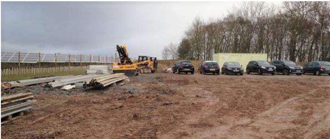
Insert 30: Start of Restoration of Construction Compound (example from Staffordshire)
