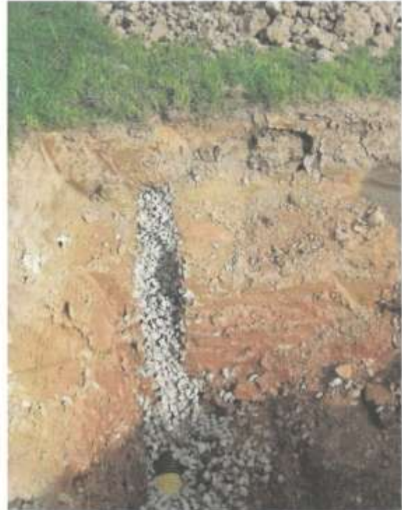
Figure 34. Permeable backfill in trench over drain
