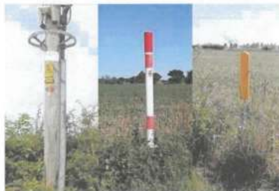
Figure 18. Signs indicating potential underground hazards
