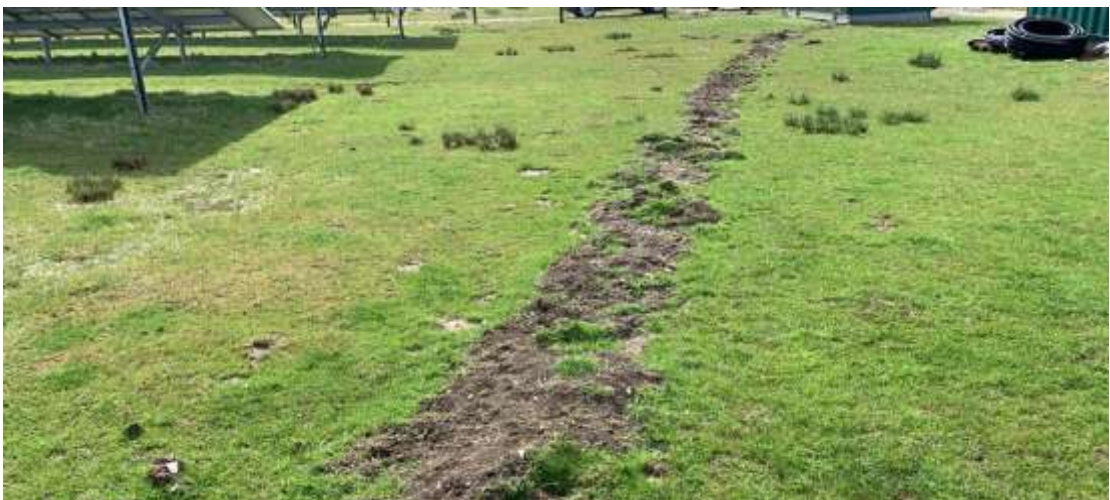
Insert 55: Trench During Wet Period
