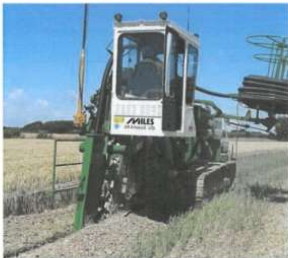
Figure 31. Installing land drains with laser gradient control
