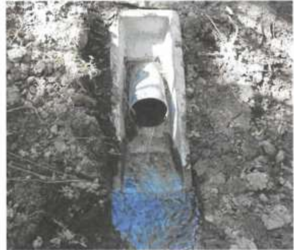
Figure 38. Precast concrete headwall (type K)
