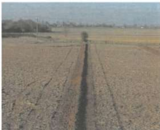
Figure 29. Recently installed drains
