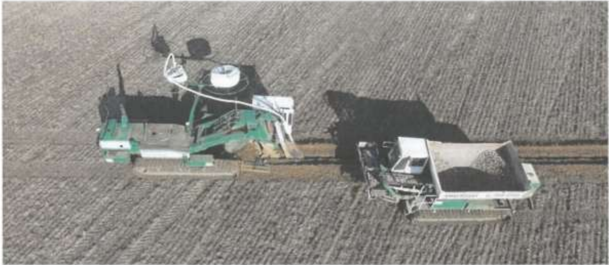
Figure 28. Installing land drains and stone backfill
