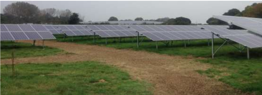
Insert 25: Localised Repairs (Solar Farm in Sussex)
