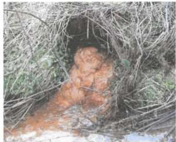
Figure 24. Drainage outfall blocked by ochre
