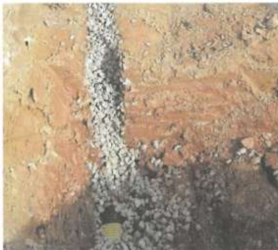
Figure 37. Washed gravel permeable fill over drain
